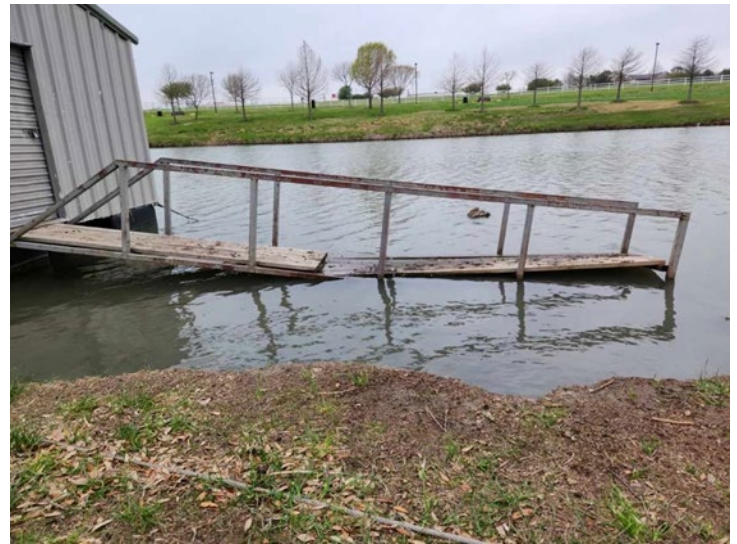
Capp Smith Park boathouse gangway
