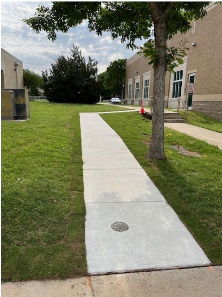
Grading around new sidewalk and laying sod
