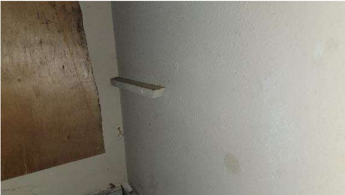
Drywall, wall texture (2% Chrysotile), and joint compound (2% Chrysotile)
