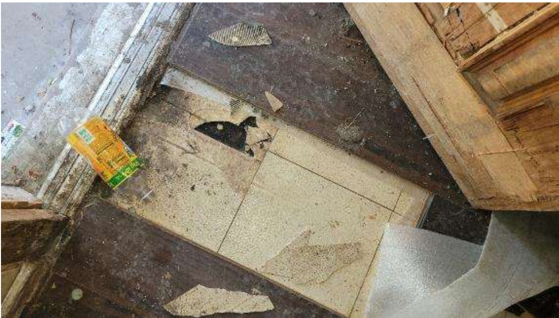
Vinyl flooring (5% Chrysotile) with mastic (7% Chrysotile)
