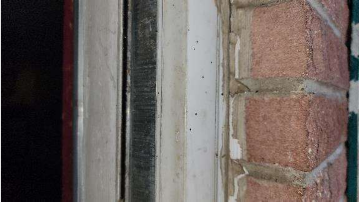
Caulking around exterior doors
